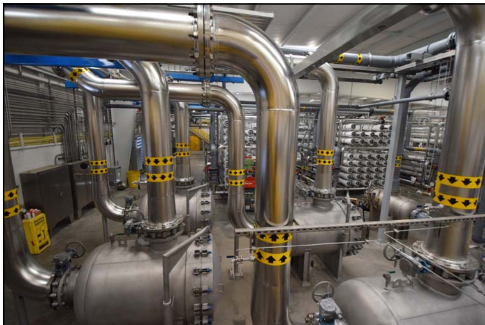
Inside Desal Production Building After Expansion Project
