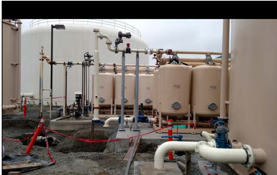
New Iron/Manganese Treatment System, Decant Tank, and Relined Chlorine Contact Tank
