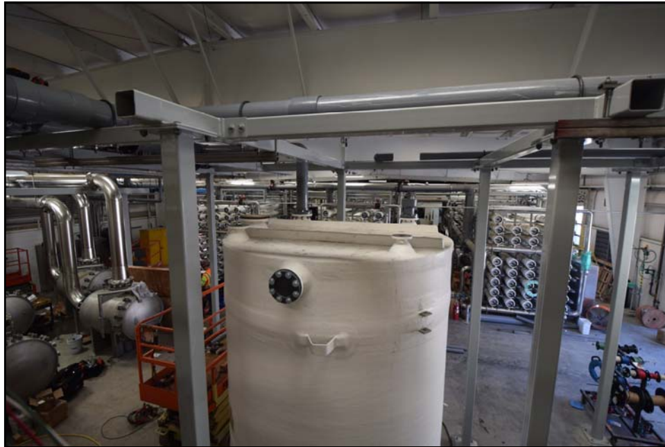
Inside Desal Production Building After Expansion Project
