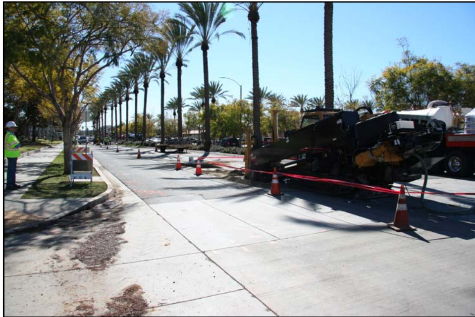
HDD Construction of 12-inch Well Conveyance Pipeline in Fourth Ave.
